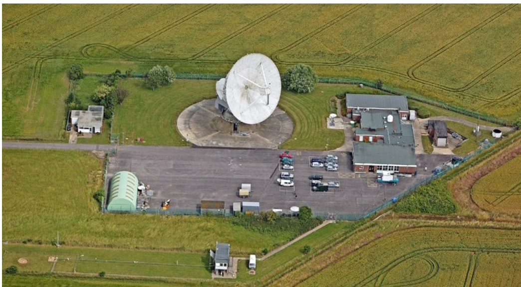
Chilbolton: View of the cloud sensing instruments alongside the 25m antenna
